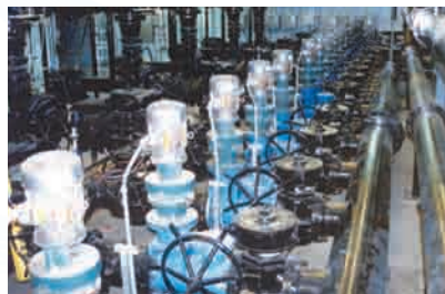
The SUPER SHREDDER in an arsenal configuration protects a major metropolitan wastewater facility.
