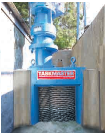
The TITAN's cutters powerfully reduce wastewater solids while allowing fluids to pass through freely.
